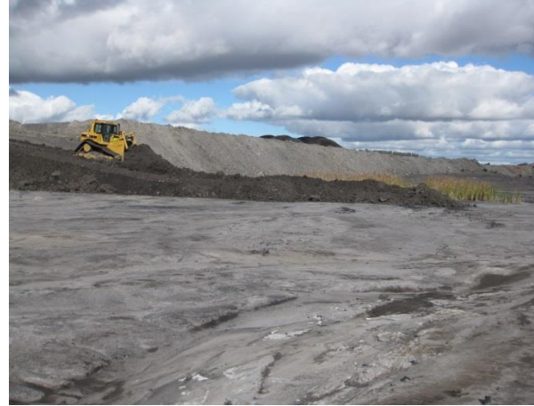
Pushing initial 1 m coarse reject capping by D6 Swamp Dozer over old bow wave
