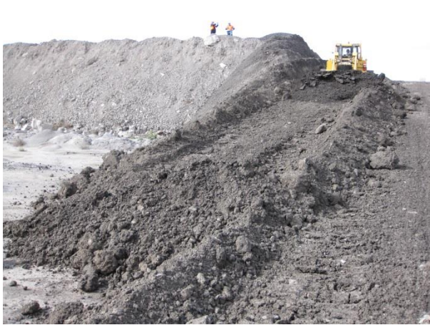
Pushing initial 1 m coarse reject capping by D6 Swamp Dozer over old bow wave
