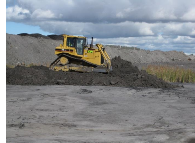
Pushing initial 1 m coarse reject capping by D6 Swamp Dozer over old bow wave
