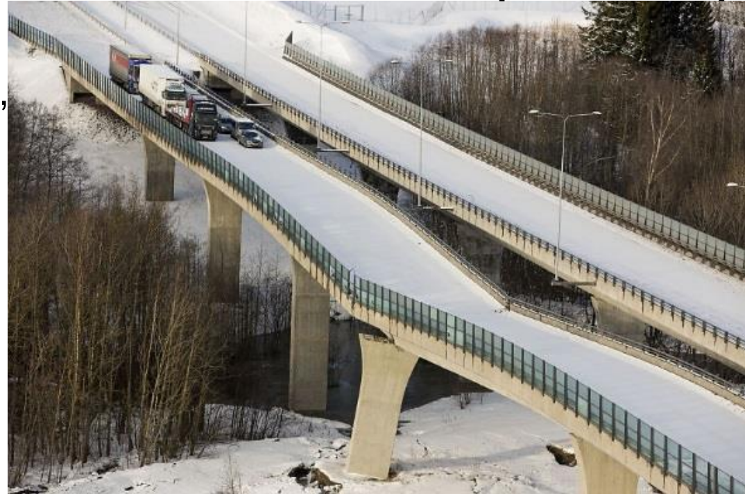
E18 expressway in Norway, February 2015 Slide in quick clay causing bridge collapse
